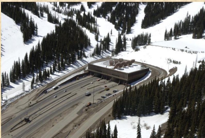
Túnel Memorial Eisenhower-Johnson
